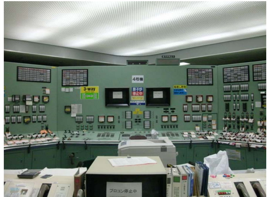
Unit 1 Main Control Room Recovery
